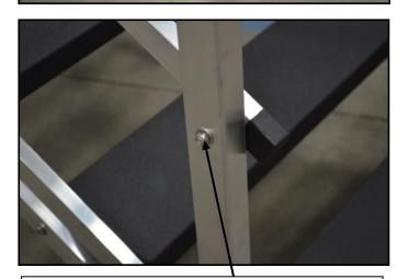
Use grease or spray lubricant on the 3/8" x 3" truss head bolts for the railing tubes. This will help prevent the stainless jam lock nuts from seizing on the truss head bolts when using power tools to tighten the nuts.
