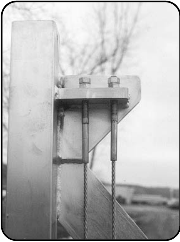
BOLT END OF OF CABLES INSTALLED. INSERT CABLES THROUGH BRACKETS. INSTALL (2) BRASS NUTS TO SECURE & LEVEL.
