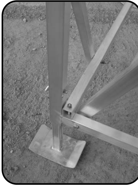
FRONT CORNER ASSEMBLY SHOWING DROP LEG, FRONT TUBE AND FRONT BRACE
